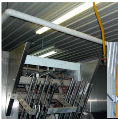
Below: Technician Matt Smith installs piping, coated yellow to indicate it is a gas line.
